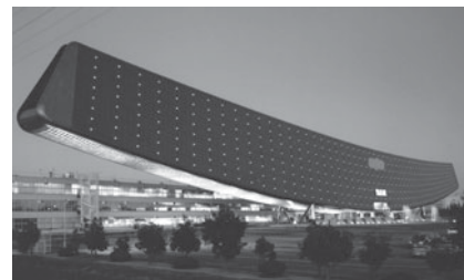
FIGURE 37.20 Japan's Sanyo Solar Ark incorporates some 5000 photovoltaic panels and generates a peak power of 630 kW.
